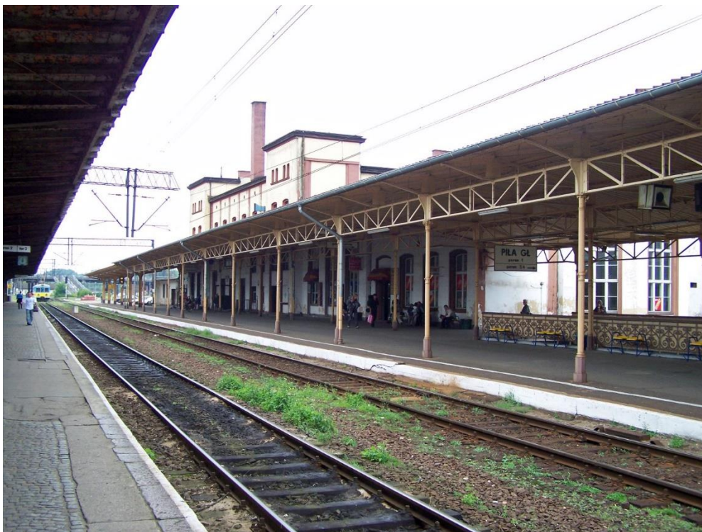
Piła's main train station
